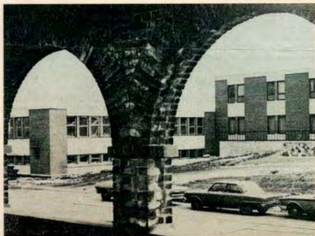
Old arches, now gone, frame this view of the new school. Wrecking of the old building began in mid-June following an "auction" on two successive Saturdays to dispose of the mementos of an era.
